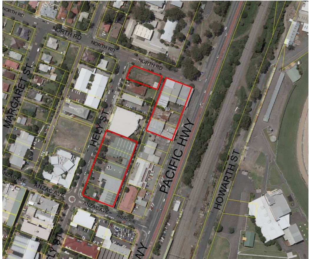
Figure 17: Aerial photograph of Anzac Avenue Community Facility and Aldi Site, Wyong
